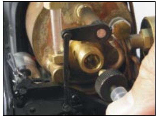
fig. #18 Attaching butane hose to boiler
